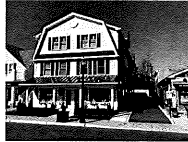
RESIDENTIAL DEVELOPMENT POSES CHALLENGES WITH PARKING, ACCESS, AMENITIES, MASSING & YEAR ROUND OCCUPANCY
